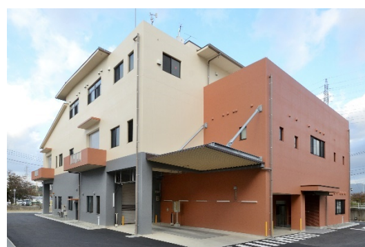
Utsugien (sludge recycling and treatment facility); Koga City, Fukuoka Prefecture
