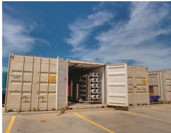
Movable containerized desalination plants
