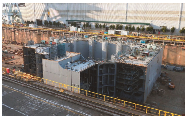
Floating bodies being produced at Sakai Works
