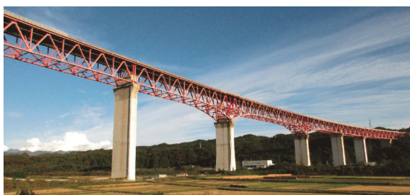
Katashinagawa Bridge (bridge length 1,034m, largest span length 169m, largest bridge column height 69m)
