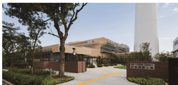
Suginami Incineration Plant
