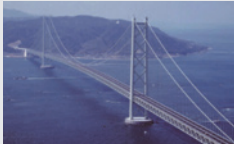
(Honshu-Shikoku Bridge Authority*, Akashi-Kaikyo Bridge) *Currently Honshu-Shikoku Bridge Expressway Company Limited
