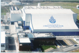
Waste to Energy plant
