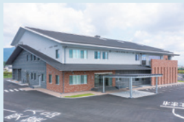
Sludge recycling center
