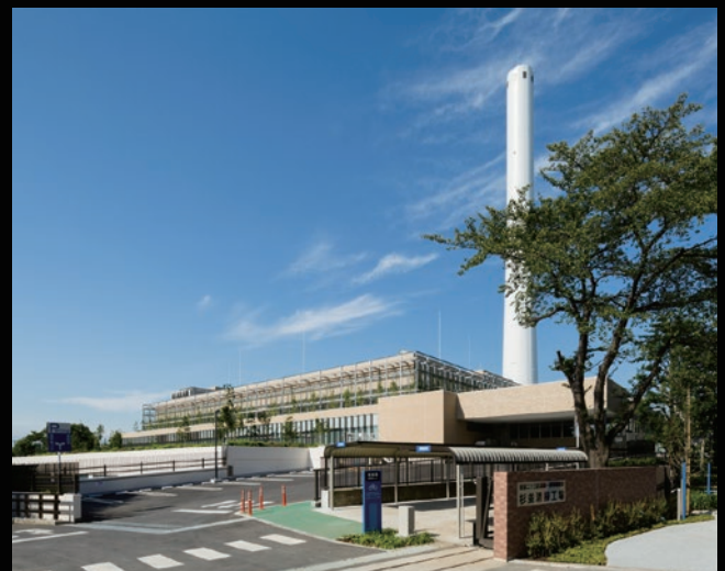
Suginami Incineration Plant of the Clean Authority of TOKYO
