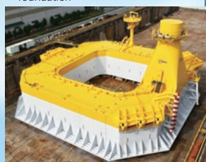
▼NEDO commissioned project: Technology demonstration experiment of a next-generation floating offshore wind turbine system (barge type); fabrication of demonstration foundation
