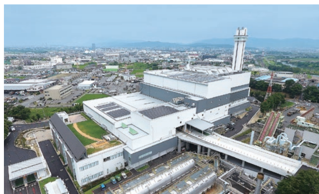
Kyoto City Nambu Clean Center
