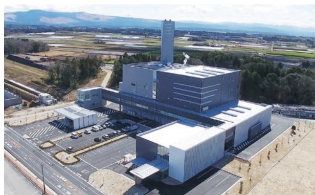
EfW Plant for Kikuchi Environmental Preservation Association
