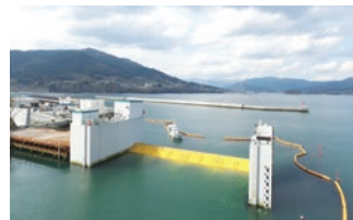
● Flap-gate type seawall against flood disaster
