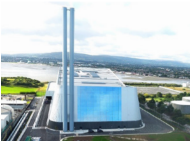
EFW plant for Ireland
