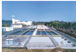
● Water and sewage treatment plants
