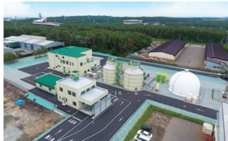
Akita Biogas Power Station
