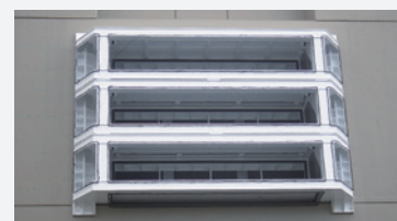
In-wall installation flap-gate type seawall against flood disaster
