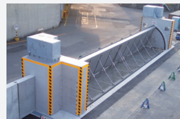
Land-mounted flap-gate type seawall against flood disaster
