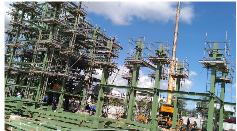
Construction site photo taken with a smart glass camera
