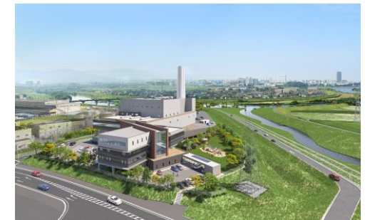
Energy from Waste plant in Saga
