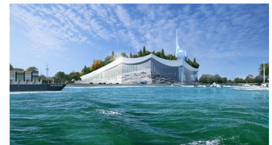
Energy from Waste plant in Shanghai
