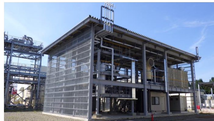
[Demonstration plant at INPEX Nagaoka field office]
