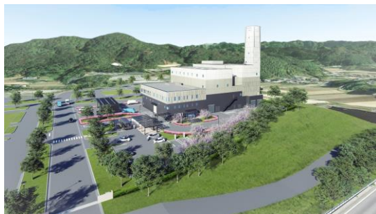
Energy from Waste plant in Uki
