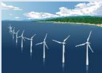
Offshore wind power generation
