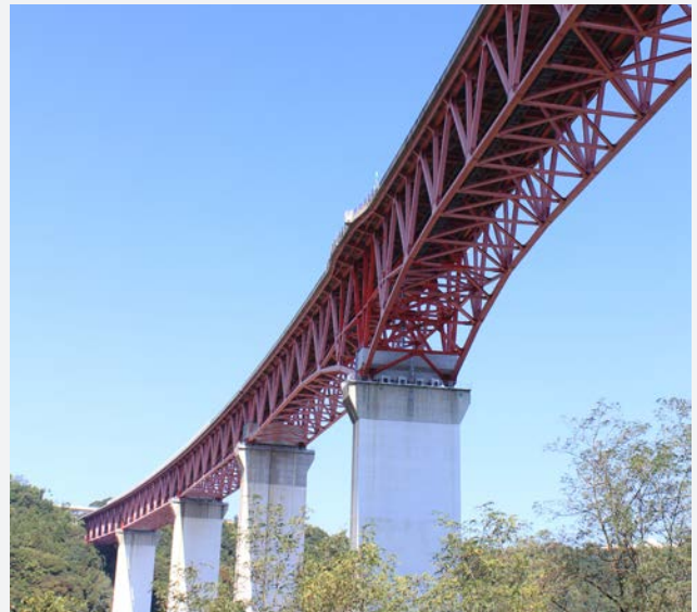
The Kan-Etsu Expressway and the Katashinagawa Bridge
