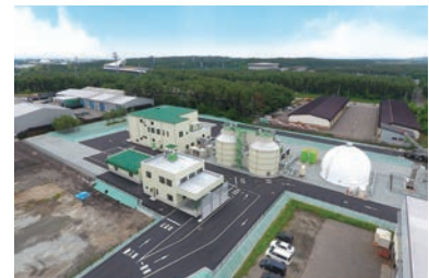
Akita Biogas Power Station
