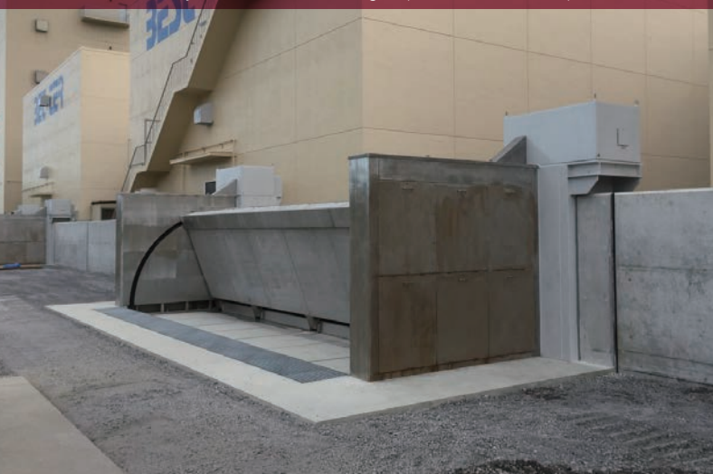
Muya Port coastal land lock gate (Tokushima Prefecture)
