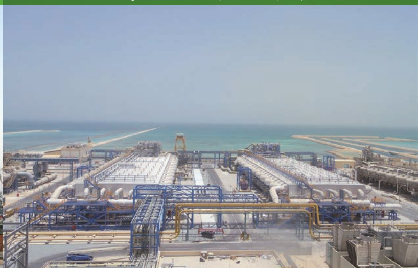
Large-scale desalination plant RAF A2 (Qatar)
