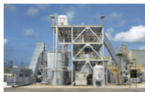
Ethanol-methane two-step fermentation system (demonstration plant)
