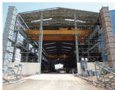
▲ New factory under construction at ISGEC Hitachi Zosen Limited
