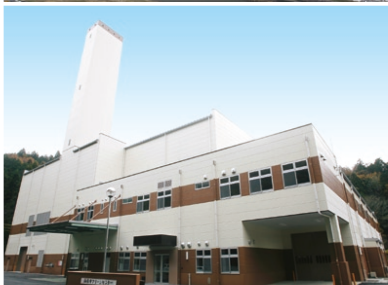
Photo: Higashiyodo Plant in Osaka City (above) Clean Center in Gifu Yamagata City
