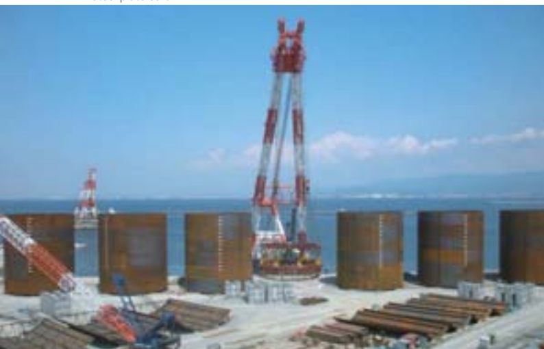
▼ Steel plate cells
