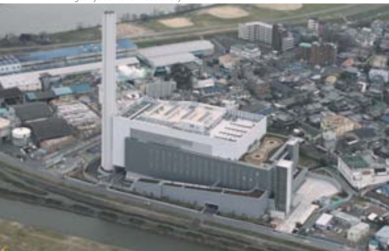
▼ Higashiyodo Plant in Osaka City
