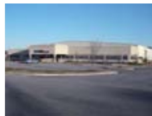
A decision was made to expand the NOx removal business by commencing operations next year at a factory run by H&N Catalyst Manufacturing LLC. in the US
