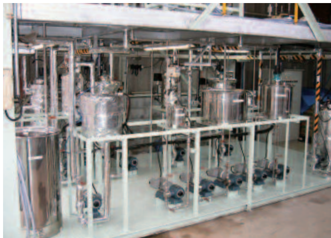
Continuous production system for biodiesel fuel
