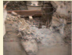
Electrical discharge shock breaker operations
