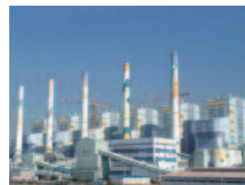
Plant installed De-NOx catalyst
