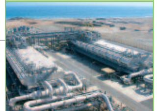
Seawater desalination plant
