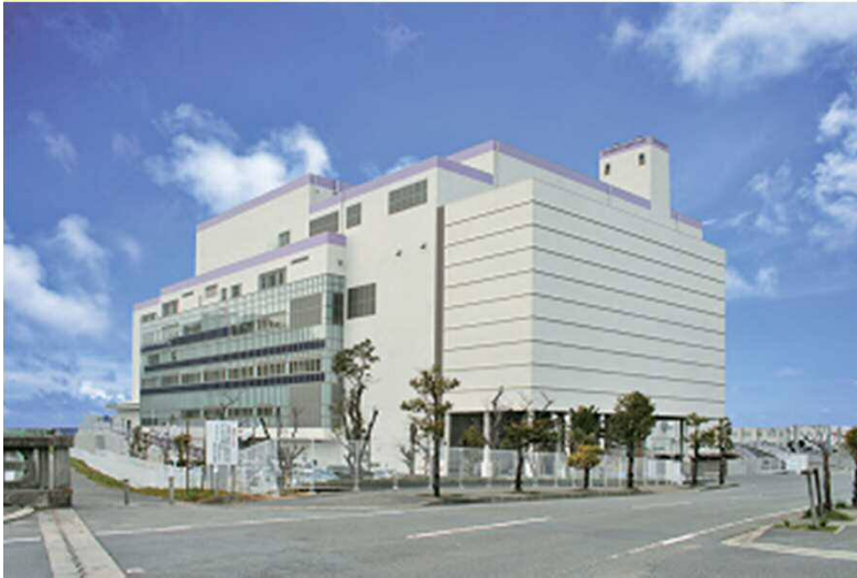
Matsuyama city shin-nishi clean center (140t/d × 3)
