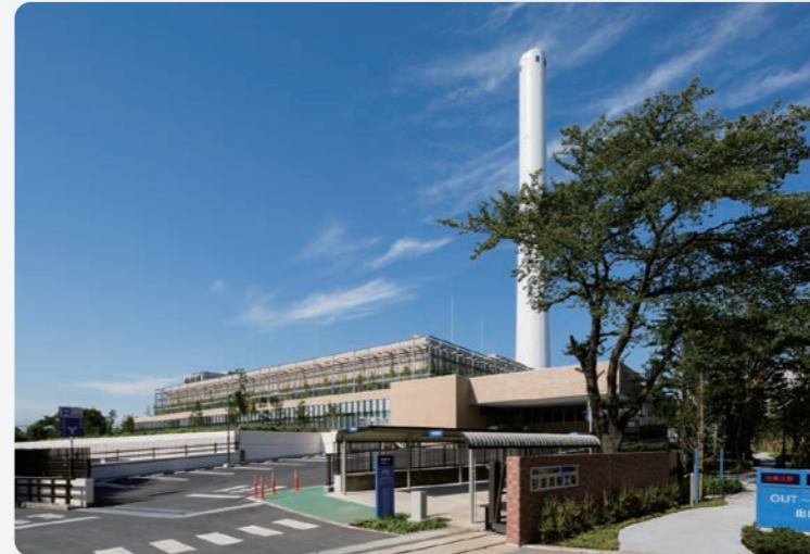
Clean Authority of Tokyo/ Suginami Incineration Plant
