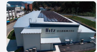
• Control Equipment Center
