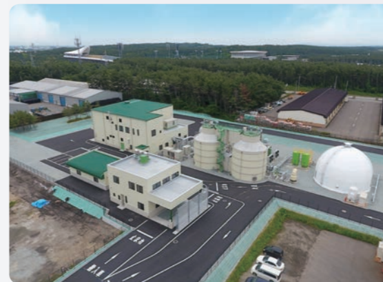
Akita Biogas Power Station
