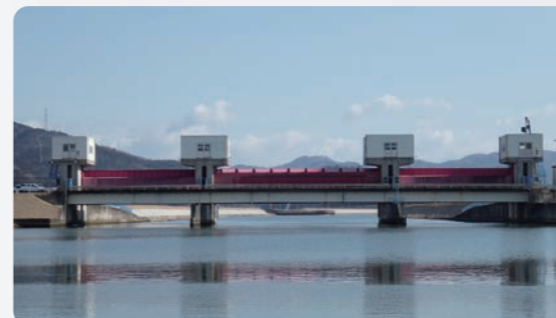
Long-span Shell Gate (Manogawa Hydraulic Gate)
