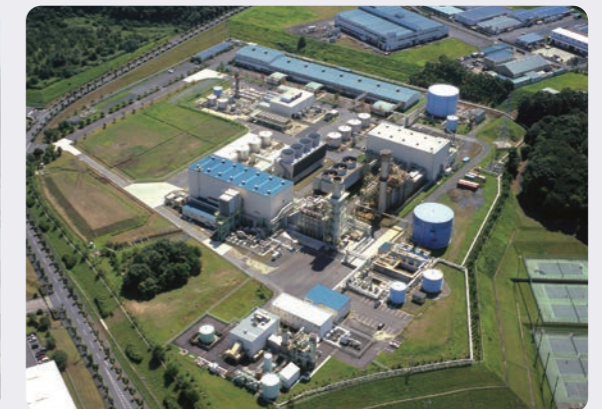
Hitachi Zosen Ibaraki Power Station
